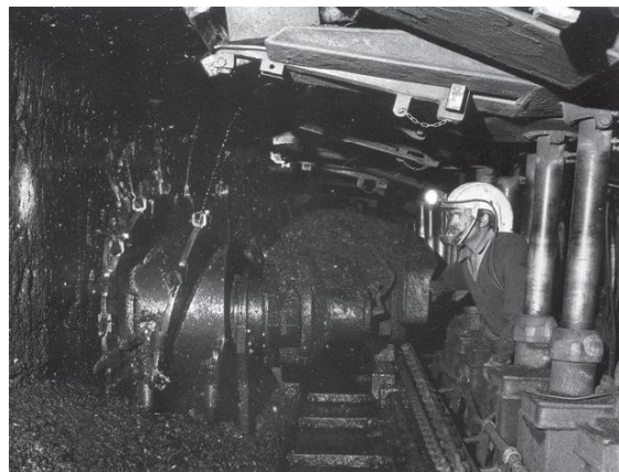
Process Control System for a Colliary
