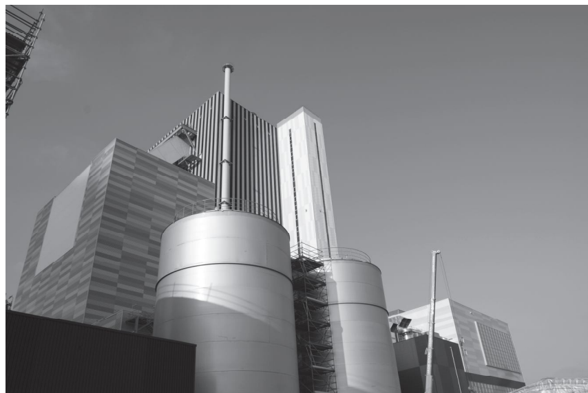
A Modern Power Plant
