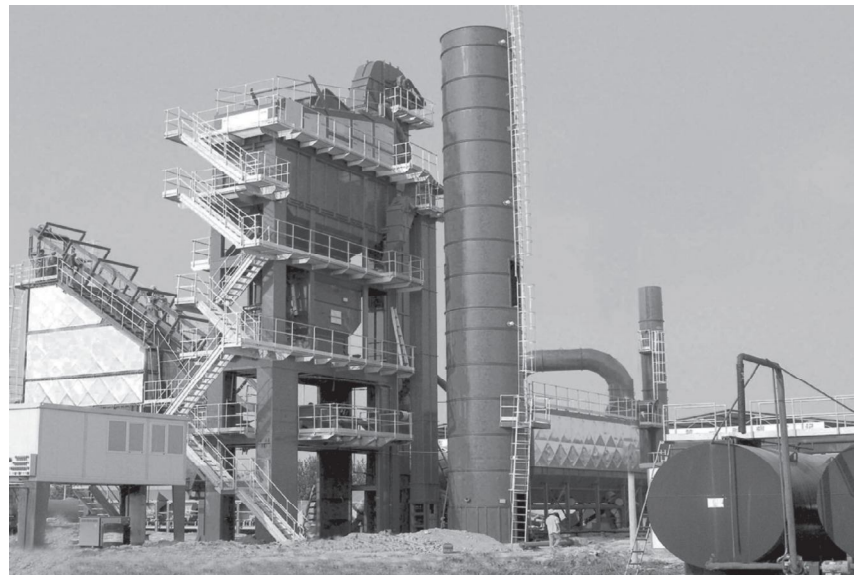
Construction site of a plant
