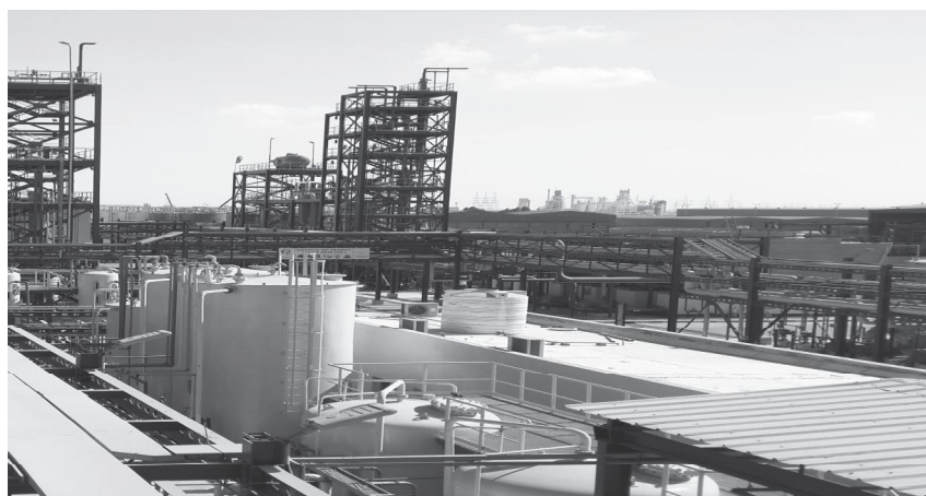
A Chemical Complex
